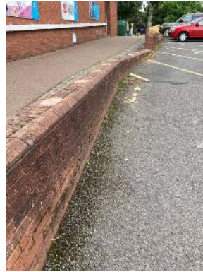
Figure 2 Low lying wall after barriers removed
